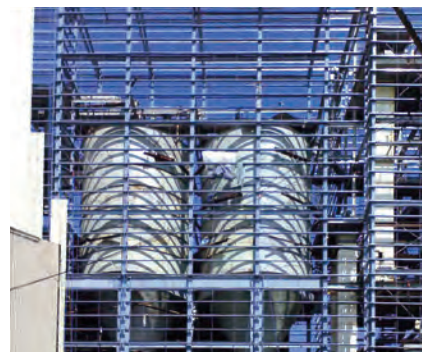
Two 500T white Sugar Silos Under Construction
